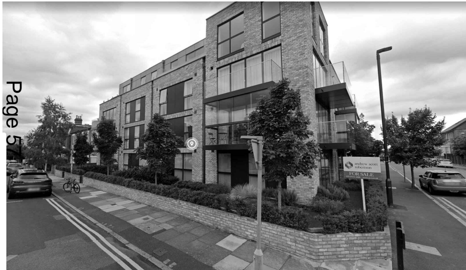
EXAMPLE WINDOW DETAIL, BRICK LINTEL DETAIL, RECESSED DOWN PIPE DETAIL & DARK GREY ZINC PANEL BETWEEN WINDOWS IN BRICK OPENING
