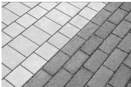
EXAMPLE PERMEABLE PAVING
